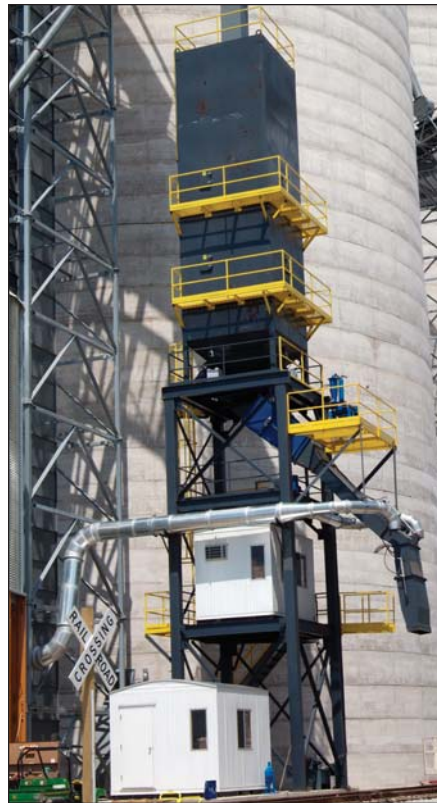
CompuWeigh bulk weigh loadout scale is designed to load a shuttle train, under normal conditions, in less than 10 hours. Ground level photos by Ed Zdrojewski.
