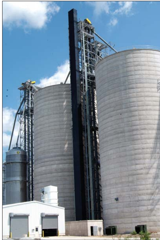
From left, dual enclosed mechanical receiving pits, two Hoffmann jumpform concrete tanks holding 500,000 bushels each, and between the tanks, two 20,000-bph Union Iron legs feeding two Union iron rotary distributors.
