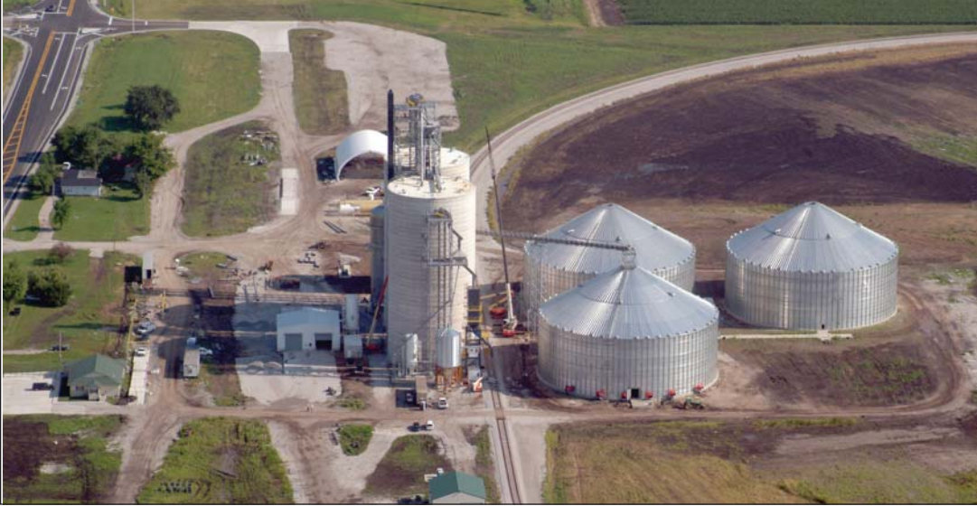
High-altitude view of the Western Grain Marketing property showing a 7,690-foot loop track for continuous rail loading without decoupling.
