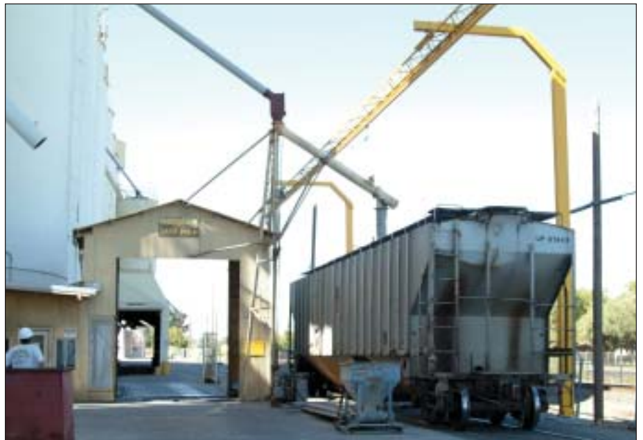
Rail unloading and loadout station at the 1030 East elevator is set up for both origin and destination weights, utilizing a bulk weigh loadout scale outfitted with CompuWeigh GMS 4000 software. Bright yellow overhead trolley unit from Fall Protection Systems protects workers atop railcars.
