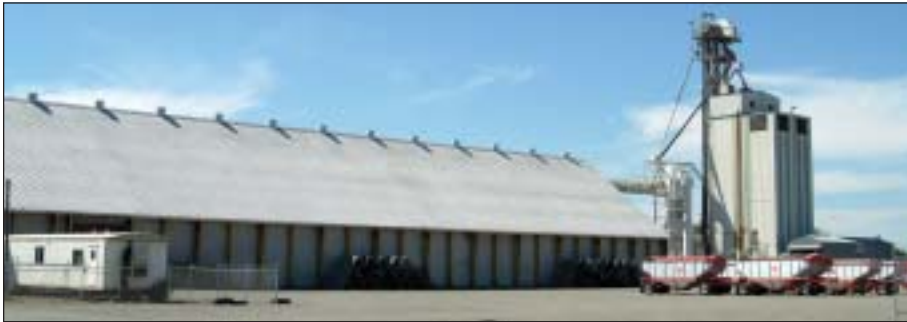
Adam's Grain Co.'s 5-million-bushel Road 102 grain elevator in Woodland, CA, includes a large flat storage building and receives and ships grain by truck. Photos by Ed Zdrojewski.
