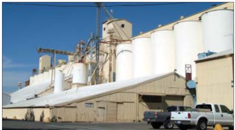
Adams Grain Co.'s 1.2-million-bushel 1030 East elevator in Woodland, CA, is a rail receiving and loading facility.
