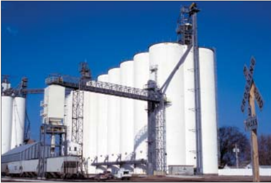
Tri-Valley Cooperative's rail terminal elevator at Monroe, NE, with two new York legs at right. Overhead 60,000-bph Hi Roller enclosed belt conveyor takes grain to a new 60,000-bph CompuWeigh bulk weigh loadout scale at left. Photos by Ed Zdrojewski.
