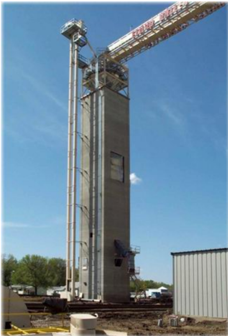
New bulk weigh scale loadout tower at Floyd Valley Grain LLC in Hinton, IA, houses a 60,000-bph CompuWeigh bulk weigh loadout scale.
