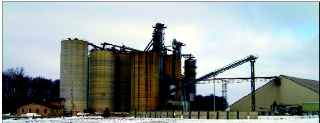
Kokomo Grain Inc.'s rail terminal in Amboy, IN, which was upgraded extensively in 2003.
