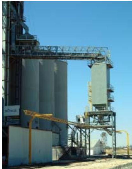
Bulk weigh loadout system installed last year at Bunge North America Inc.'s rail-loading terminal at Waterloo, IN, which includes a 60,000-bph CompuWeigh bulkweigher. Photos by Ed Zdrojewski.
