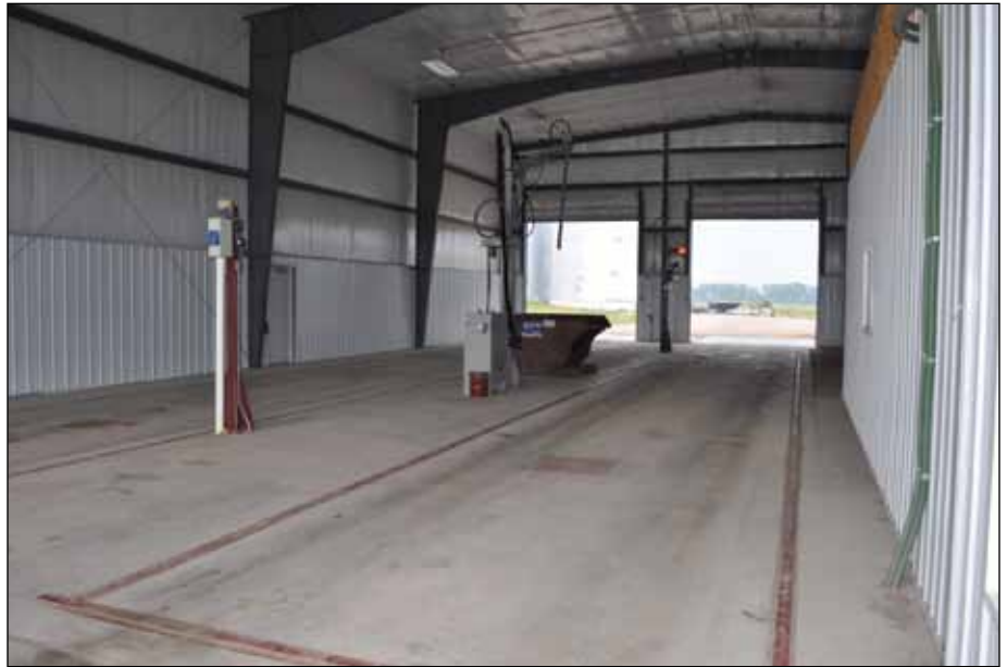
Enclosed inbound and outbound Webster truck scales are equipped with an Intersystems truck probe and a scale ticket printer.
