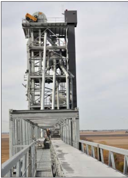
Rooftop equipment visible includes a 20,000-bph, head sections of three GSI legs, top section of a PMI (Schumacher) 650-lb.-capacity manlift, eight-hole Union Iron Works double distributor, and 20,000-bph Intersystems gravity screener.
