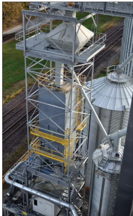
Overhead view of a 40,000-bph Intersystems gravity screener and 40,000-bph Compu-Weigh bulk weigh loadout scale.
