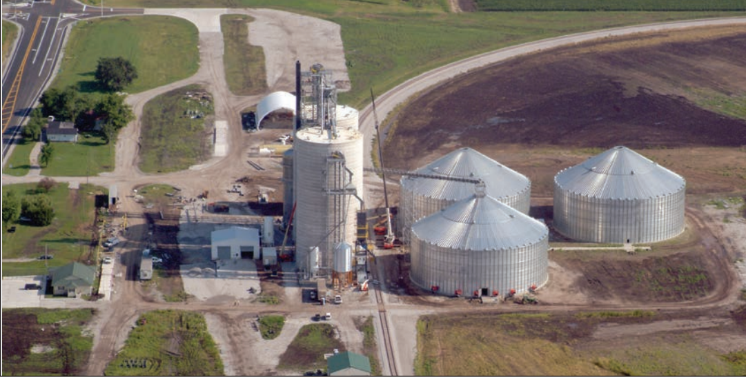
High-altitude view of the Western Grain Marketing property showing a 7,690-foot loop track for continuous rail loading without decoupling.
