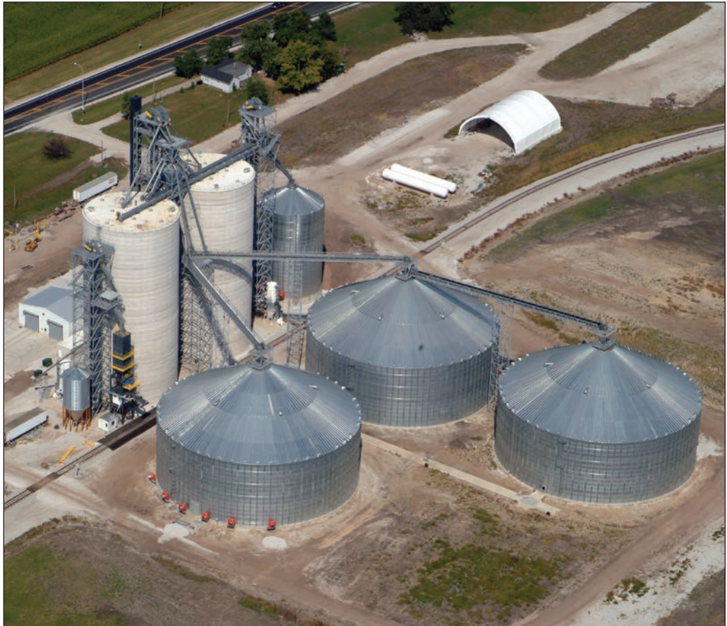
Western Grain Marketing LLC's new 4.6-million bushel rail terminal north of Adair, IL, is designed to load 110-car shuttle trains on the Burlington Northern Santa Fe. Aerial photos by B&M Studio of Photography, Pekin, IL.
