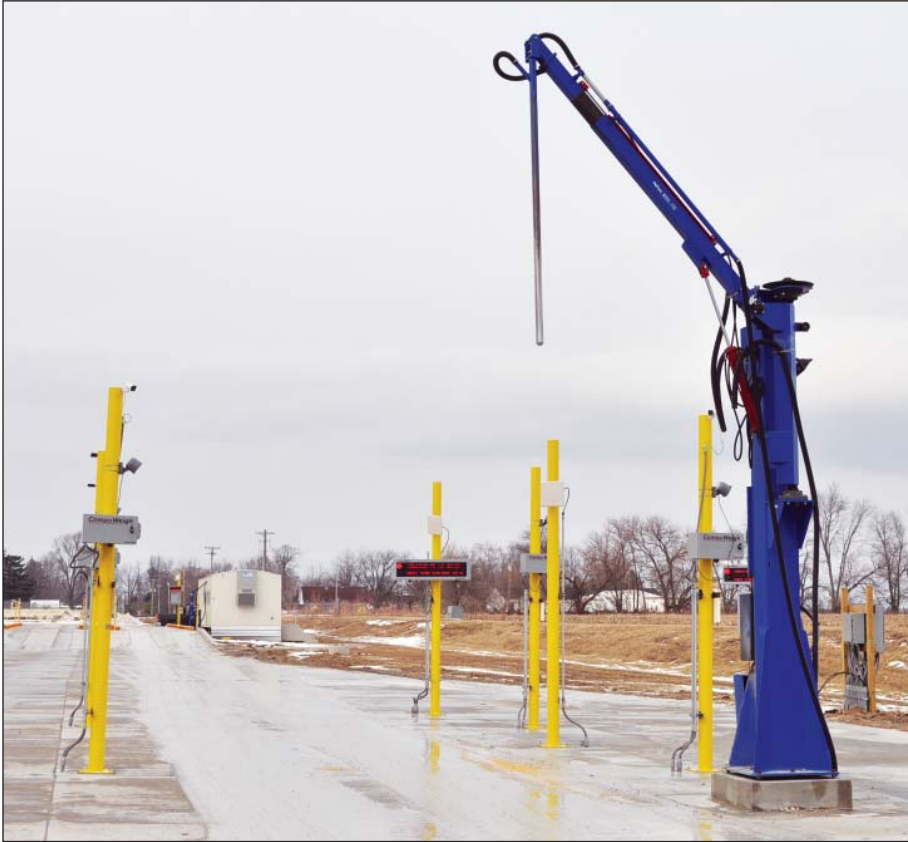
Truck receiving operations at the AC Grain rail terminal in Dana, IN, include a scalehouse, probe station, and pair of Fairbanks inbound and outbound scales, all under the control of a CompuWeigh SmartTruck automation system. Photos by Ed Zdrojewski.
