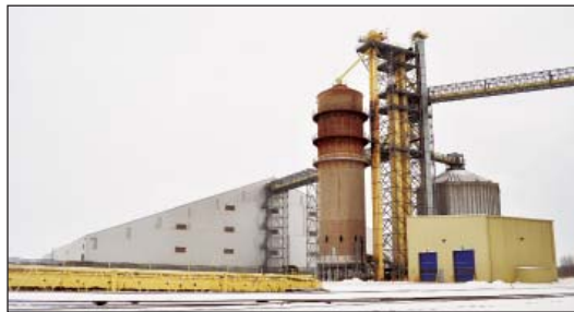
AC Grain's 9-million-bushel annex includes a flat storage building, upright wet tank, two receiving pits and legs, and a grain dryer, all of which went operational in 2013.
