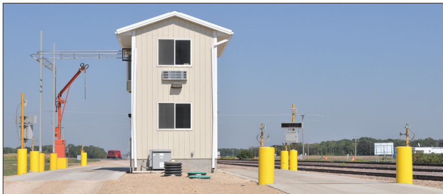
Crystal Valley Coop's upgraded truck receiving station at Madelia, MN, with two-story scalehouse and inbound and outbound scales, all tied together with a CompuWeigh SmartTruck receiving automation system. Photos by Ed Zdrojewski.
