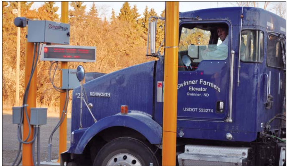
Driver awaits instructions from a CompuWeigh SmartView message board on where to deliver his load at a Full Circle Ag grain terminal in Forman, ND. Truck receiving operations are now under the control of a CompuWeigh SmartTruck automation system. Photos by Ed Zdrojewski.
