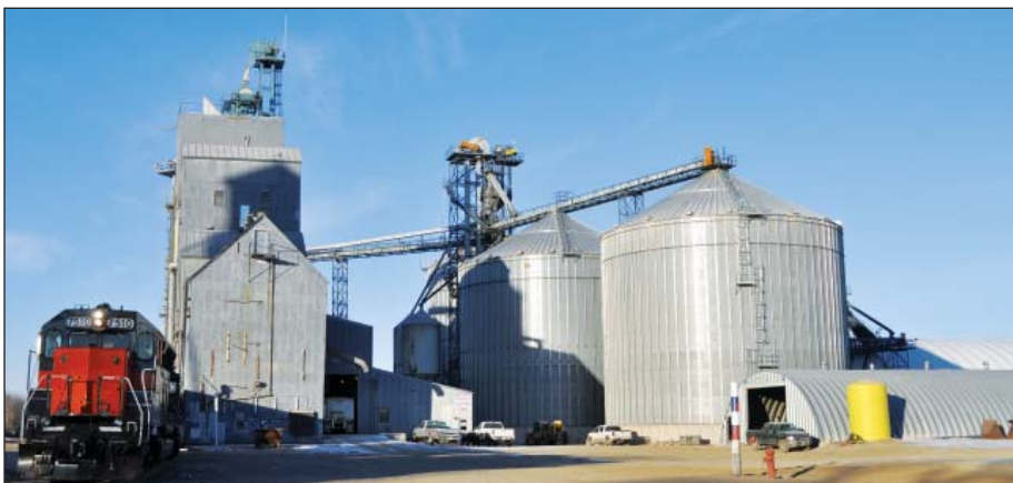
Full Circle Ag's rail-loading elevator at Forman, ND has 1.2 million bushels of storage capacity and loads trains on the Canadia Pacific.
