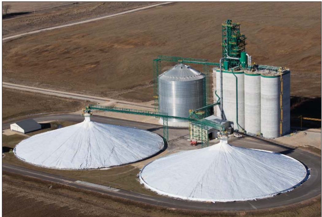
4.6-million-bushel rail terminal at Fall River, WI includes slipform concrete and steel upright storage and two temporary storage piles. Photos by Ed Zdrojewski.
