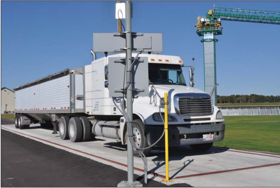
Incoming grain truck is weighed on an 80-foot B-TEK pit-type scale under the control of a CompuWeigh SmartTruck automation system.
