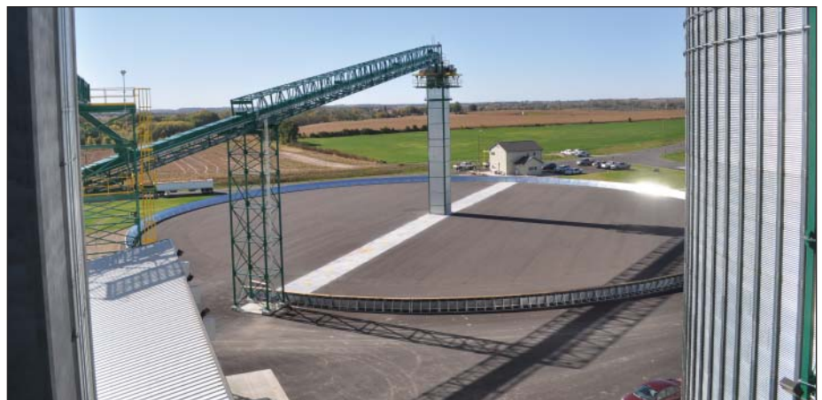
One of two 1.5-million-bushel temporary storage piles with LeMar center fill tower. This one also has a below-ground Hi Roller 20,000-bph reclaim conveyor.
