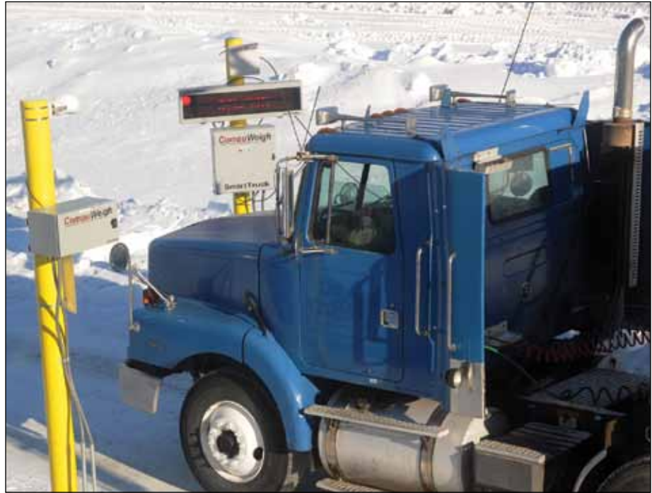
A driver waits for the CompuWeigh SmartTruck system to release him from the scale while hauling a load of grain to Maple River Grain and Agronomy, LLC in Casselton, ND. SmartTalk intercom at left allows driver to speak to office staff. Photos by Robb Siverson Photography, Fargo, ND.
