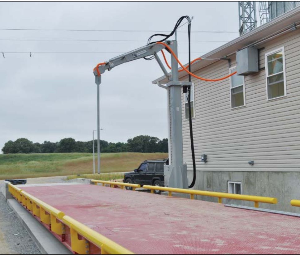
Rice Lake pitless inbound-outbound truck scale and InterSystems truck probe adjacent to the facility office building and grain lab.
