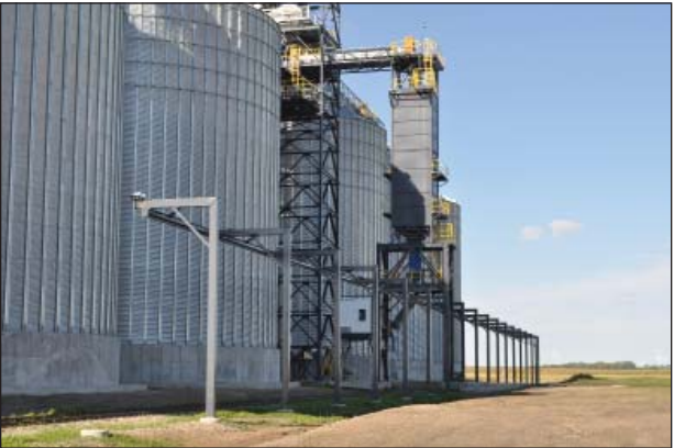
An 80,000-bph Warrior bulkweigher is used to load shuttle trains. The trolley-type fall protection unit, fabricated by Warrior, runs for 500 feet.
