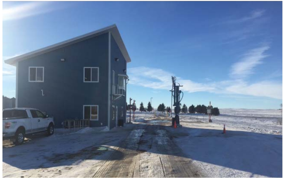
New receiving building, truck probe, and inbound truck scale operated by Finley Farmers Grain & Elevator Co. south of town. Photo courtesy of CompuWeigh Corp.
