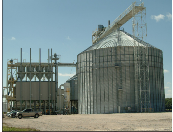
A new, 1.55-million-bushel steel bin will be built at Aurora West by Behlen Mfg. Co. adjacent to this 550,000-bushel grain tank.
