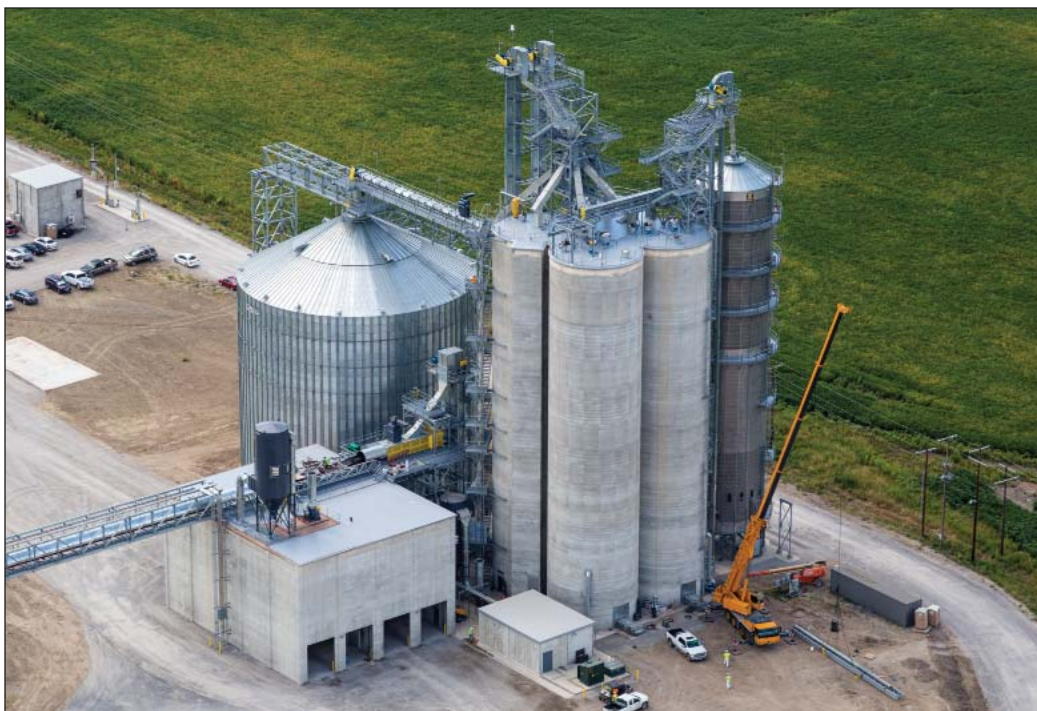
Louis Dreyfus Company's new 800,000-bushel river terminal at West Memphis, AR sends grain more than half a mile via covered belt conveyor (left) out to moored barges. Photo by Aerial Innovations of Tennessee, Nashville.
