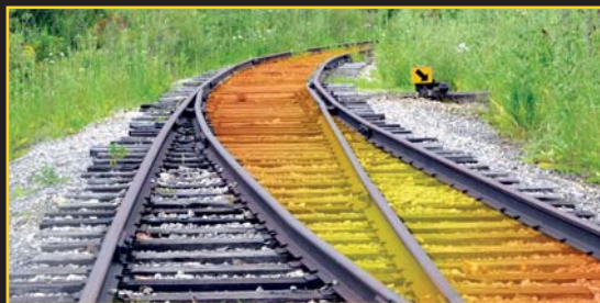
frog end of switch lined for left turnout
