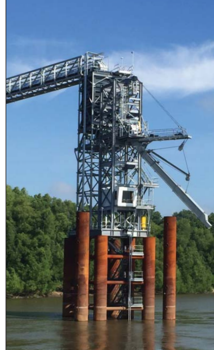
Warrior stair tower over the water supports a Warrior/Micada surge bin and a Premier Fabrication loadout spout. A covered belt conveyor running more than half a mile in a Warrior box bridge brings grain from the elevator. Photo from Louis Dreyfus Company.
