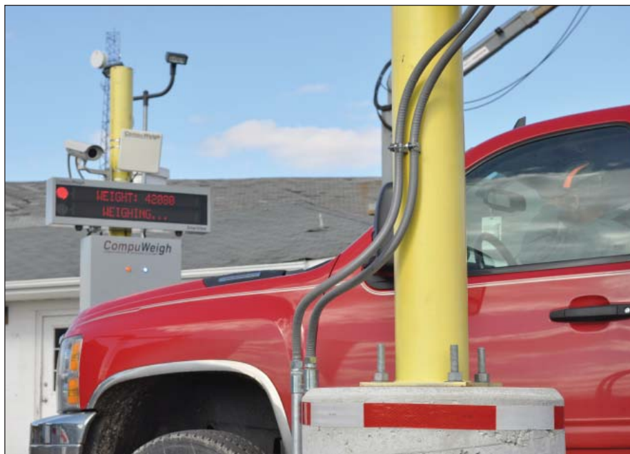
CompuWeigh SmartView digital display monitor directs a driver to the correct receiving pit, part of the SmartTruck traffic automation system at Sunrise Cooperative in Sidney, OH. Photos by Ed Zdrojewski.
